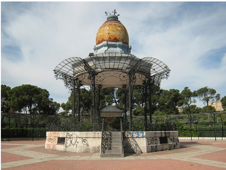
Zaragoza. Bandstand for the Hispano-French Exhibition, 1908. Use of cast-iron columns.
